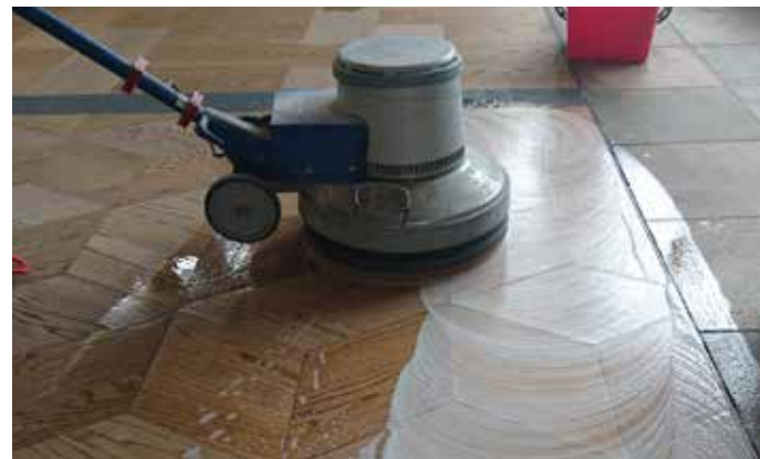
► Fig. 3 Rubbing with a polishing machine
